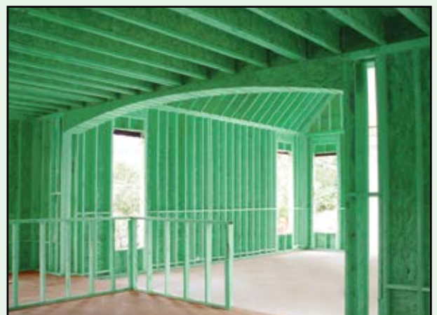
There is only one chance to install mold-resistant wood: when the home is built.
